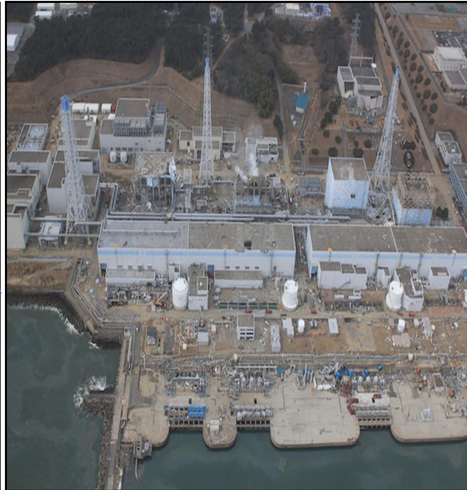
After the Earthquake and Tsunamis
